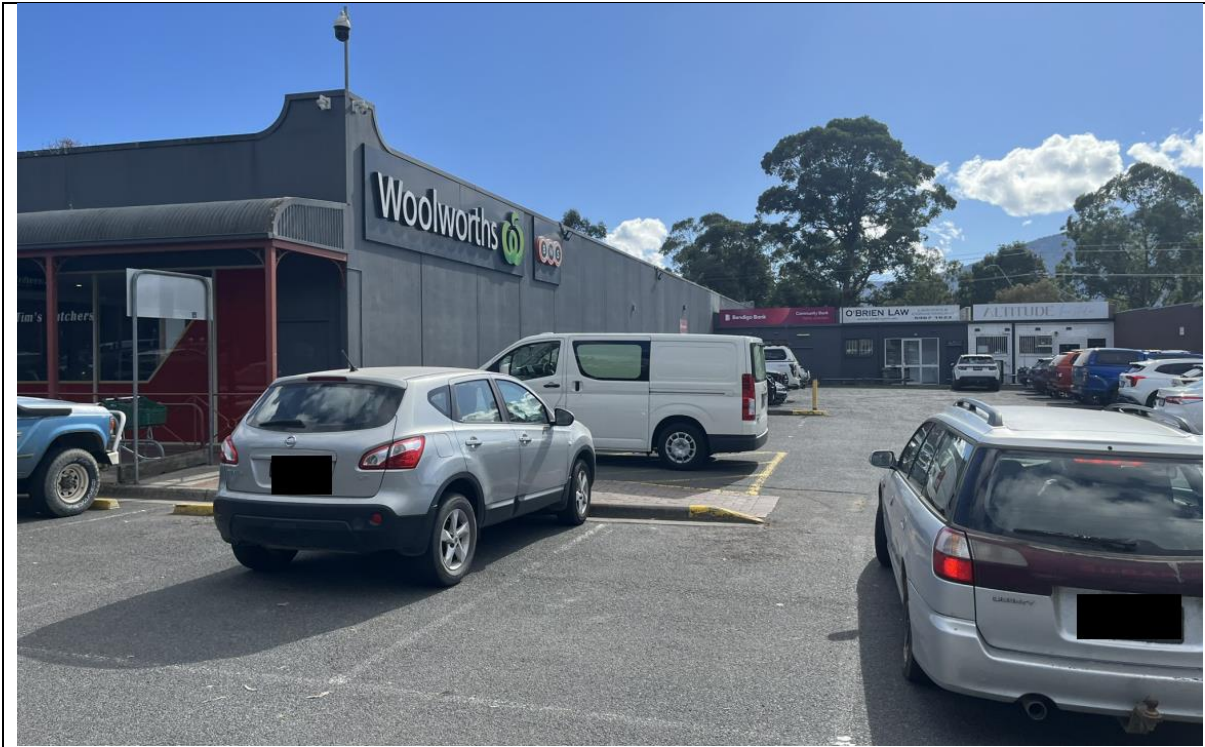
Photo 5 – South elevation area of extension
