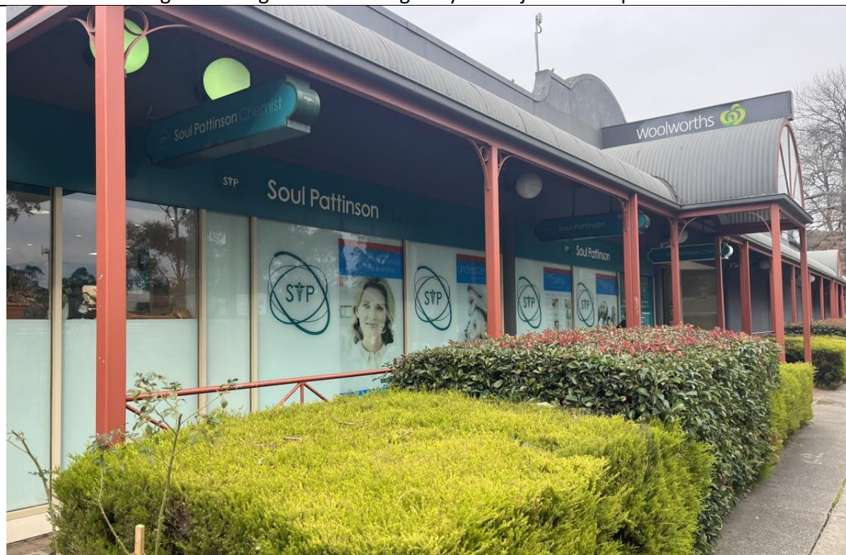
Photo 2 – Subject development – North Elevation
